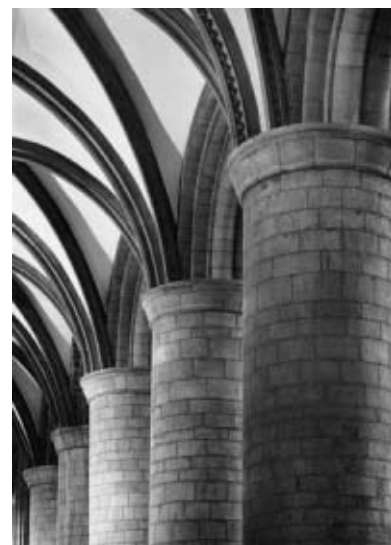
B. Piers, Gloucester
