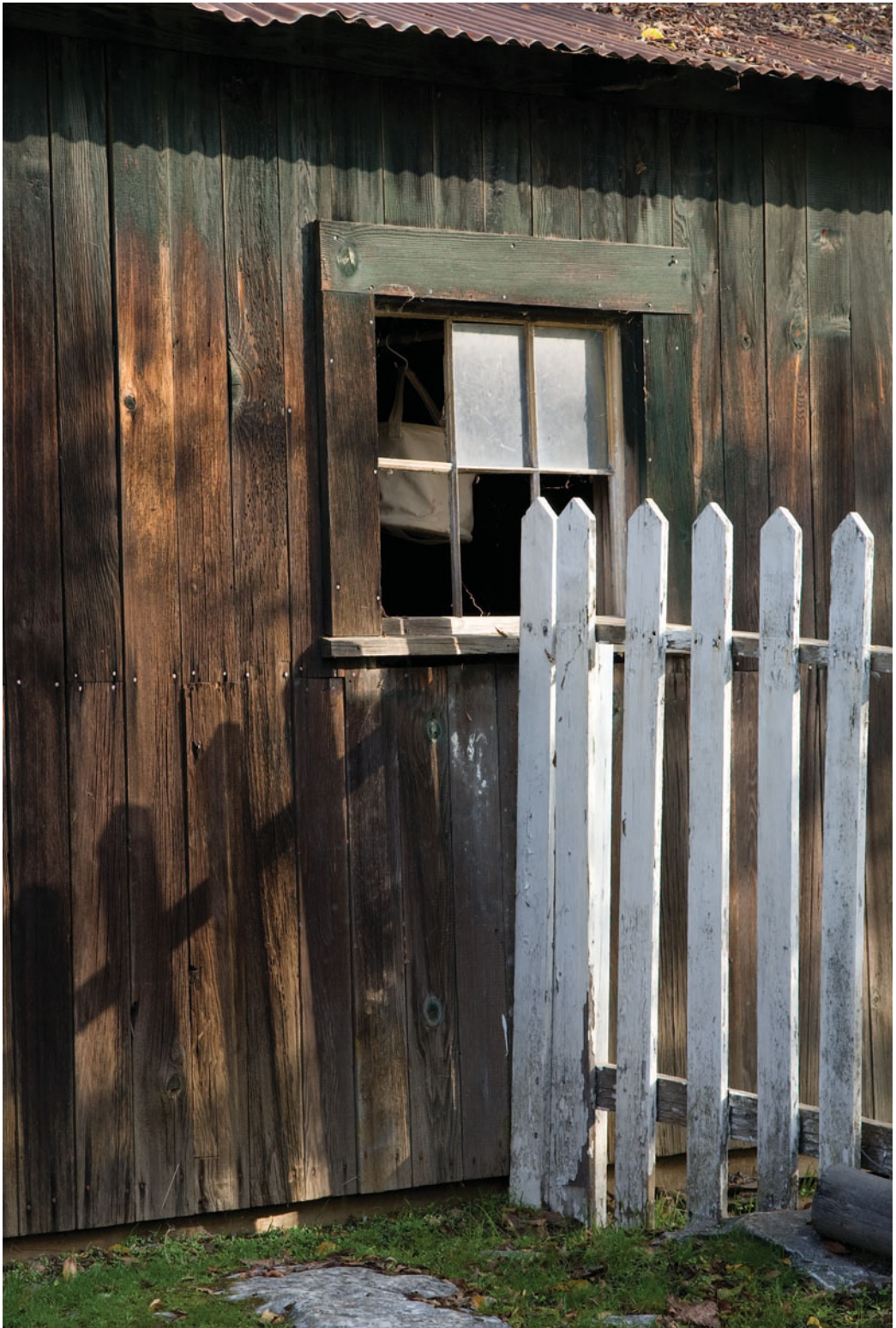
Old building in Columbia, California.
