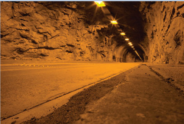
The tunnel is asymmetrical.
