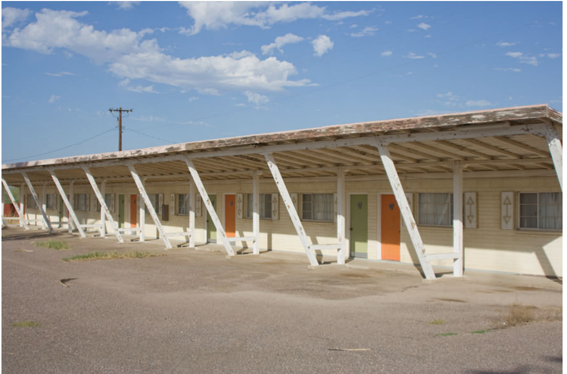
Abandoned motel in Arizona.
