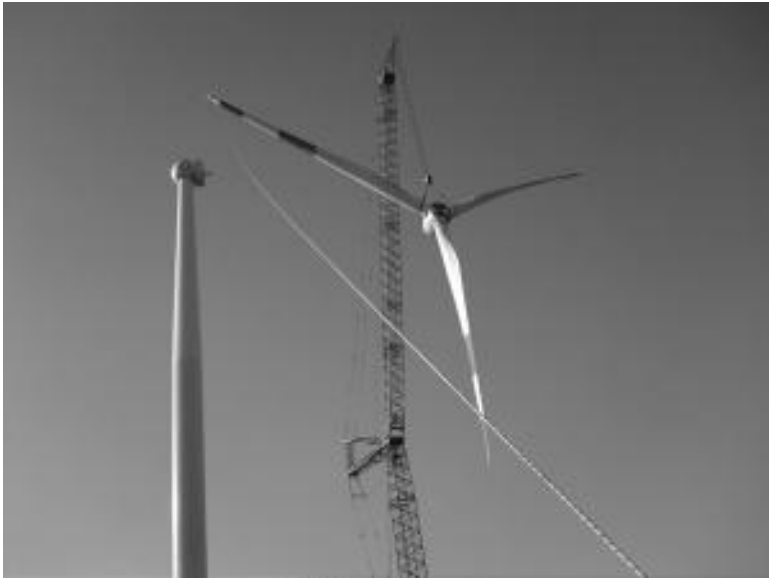
FIGURE 14-6 Main 500-t crane lifting the rotor assembly of 1.5-MW Vensys 77, 100-m hub in Nuekirchen wind farm near city of Eisenach in Thuringen Germany. Ropes are tied to the two top blades to ensure that it does not hit the tower. (Courtesy of Vensys Energy AG).
