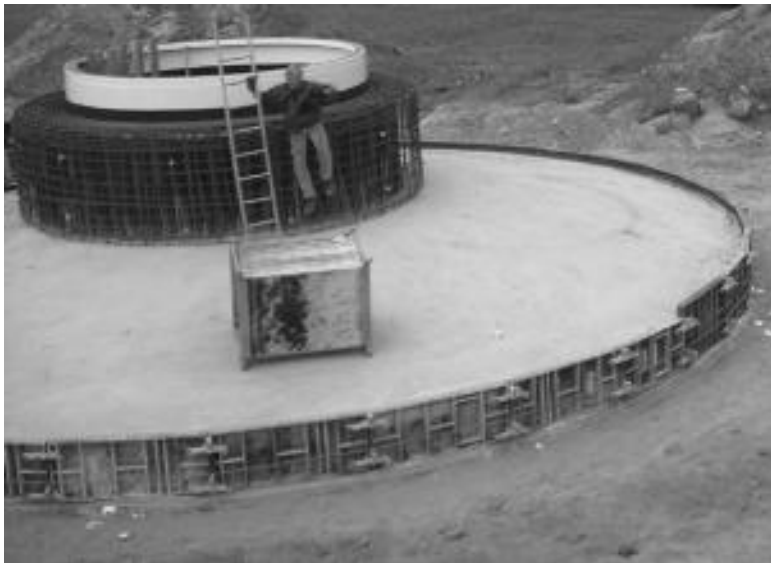
FIGURE 14-4 Spread foundation after concrete has been poured in the footing of the foundation. (Courtesy Vensys Energy AG.)
