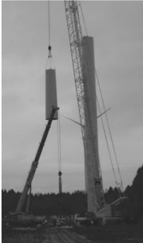
FIGURE 14-5 Lifting of tower sections by the main crane (right). Auxiliary crane (left) assists with the lift. (Courtesy Vensys Energy AG.)
