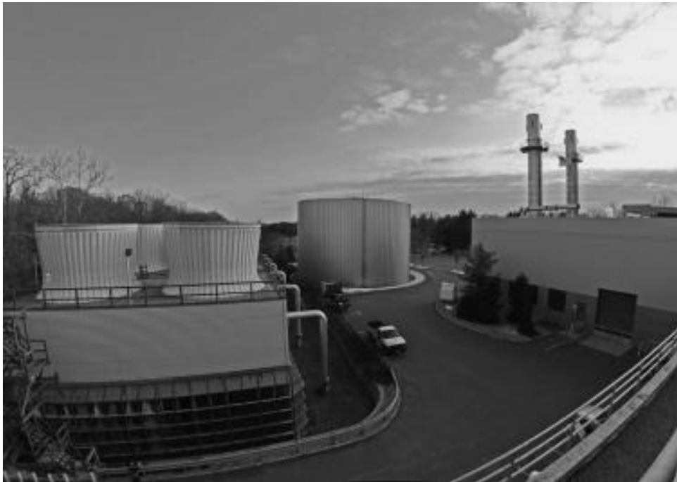
FIGURE 19-1 View from Princeton's energy plant roof. ( Courtesy of Christopher M. Lillja. )
