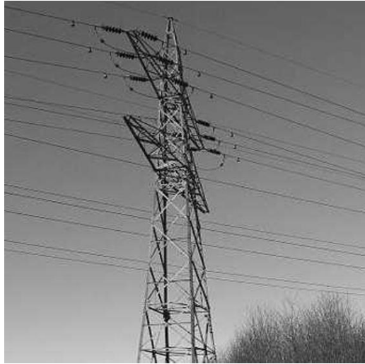
Figure 1. Pylon, a typical example of a truss
