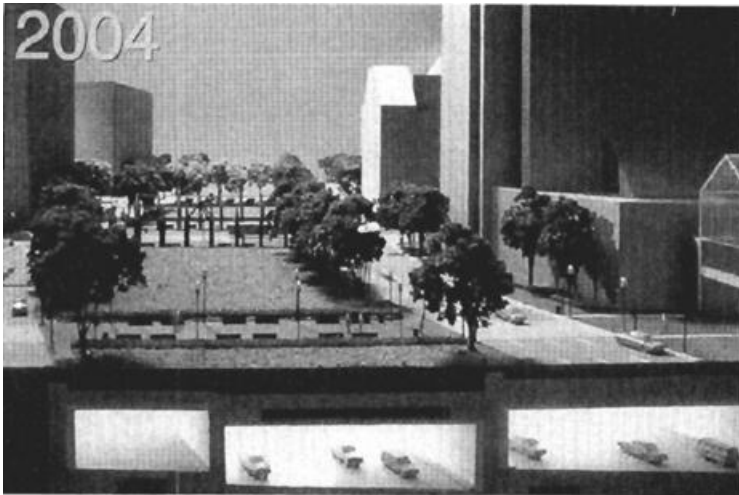
A SECTION OF THE FUTURE UNDERGROUND ARTERY BENEATH THE DOWNTOWN AREA, CLEARED OF THE ELEVATED ARTERY, IN THE YEAR 2004. (Courtesy Central Artery/Tunnel Project)
