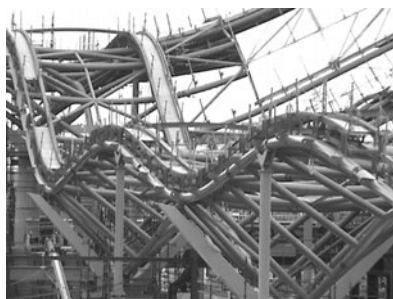
Figure 1. An application of functions to the roofing structure at Southern Cross Railway Station, Melbourne
