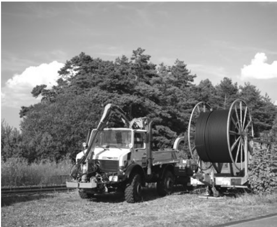
Figure 1. Usage of a cable drum in road work (copyright ©Helga Lade)
