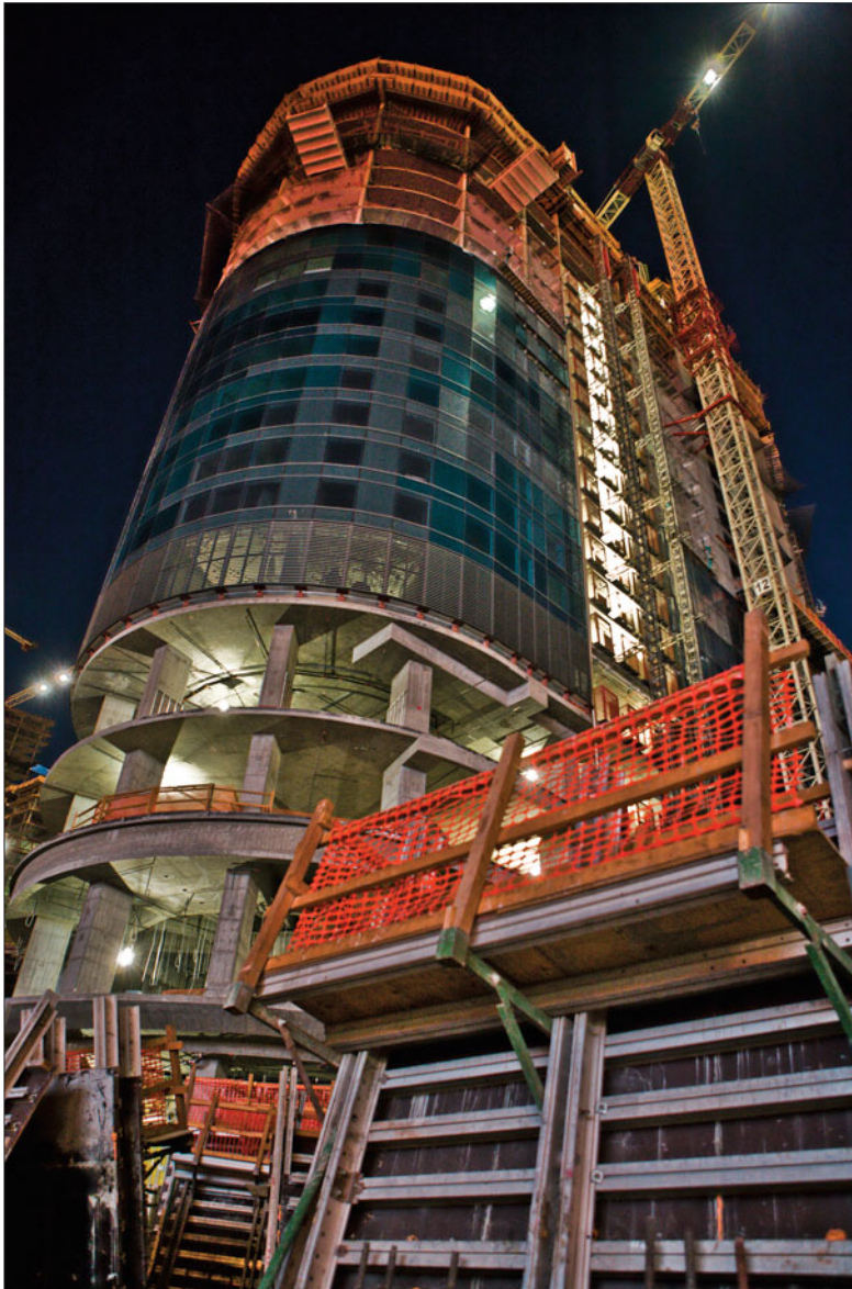
Figure 3.11 Construction site, Las Vegas, Nevada—You can often open up for night scenes that include light sources. f2.8 @ 1/40, ISO 1600
