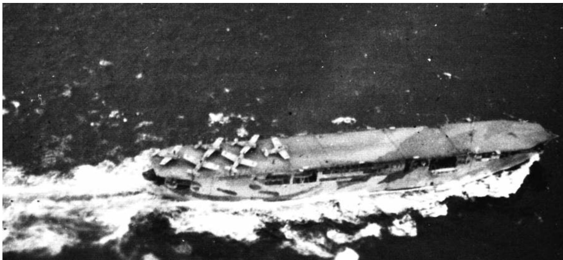
HMS Audacity with six Martlet fighters on deck, late 1941. The lack of an elevator meant that all maintenance had to be carried out on deck and the aircraft were constantly exposed to the elements.. (Author's collection)
