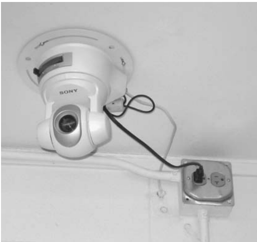
FIGURE 1-4 Avoid exposing power and data cables, providing an easy method of disabling the security camera.
