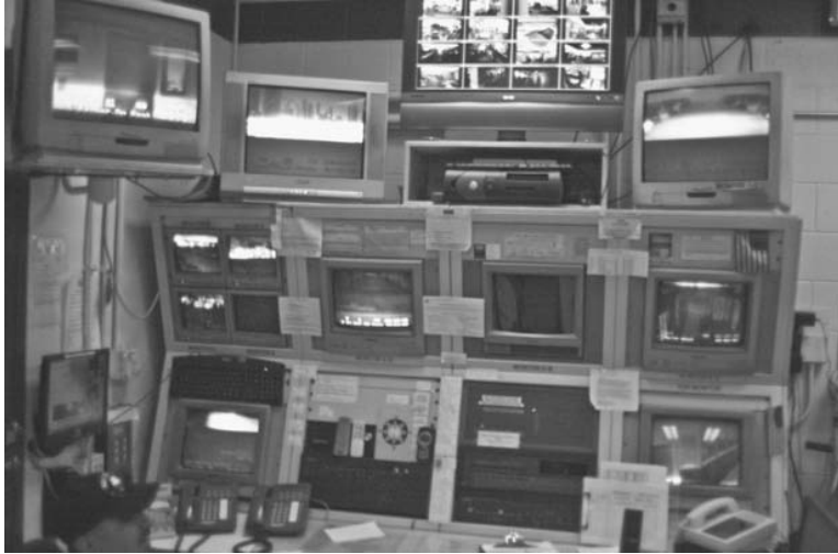
FIGURE 7-2 Before the DVS convergence there were many separate video surveillance and alarm systems running on multiple interfaces ( photo courtesy of IBM and Navy Pier ).
