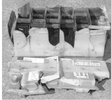
FIGURE 7-24 Battery explosion resulting from gassing.
