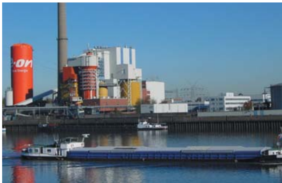
Figure 2. The location of the Farge plant allows for the co-combustion of sludge from the adjacent sewage works with the supply of coal brought in to the plant's own dock
