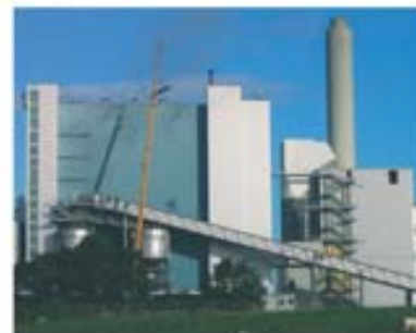
Lanesborough, Ireland, 100 MWe 414.000 m 3 /h, Dry CFB FGD
