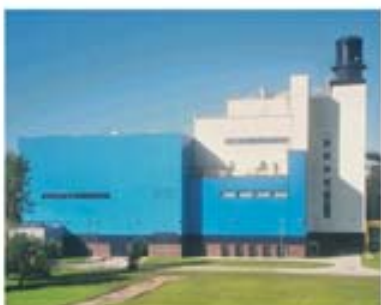
CCPP Lublin, Poland, 235 MWe
