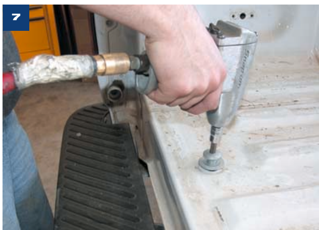
7 Anchor bolts fastening the truck bed to the truck frame are removed so spray-in material coverage is complete.
