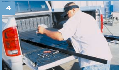
The framerrails, drip trail, strike loops, and hardware is gathered in the truck bed in preparation for the installation.
