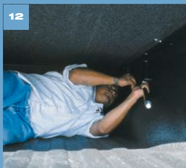
The installer then rechecks the hinge in the hinge pocket and tightens all loose hardware.
