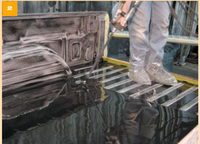
Once that area has dried, the second stage is poured on thick and will fill the area to make the bed floor flat.
