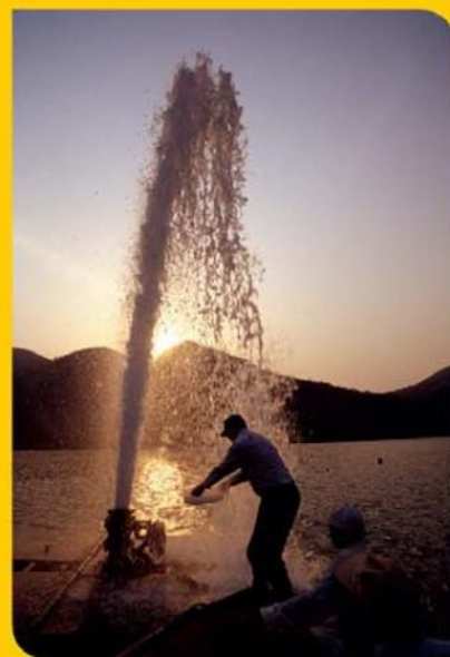
Pumps in Lake Nyos in Cameroon will reduce the gas content in the lake.
