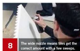
7 UA's own 'Space Mist' adhesive proved ideal to mount their tiles.
