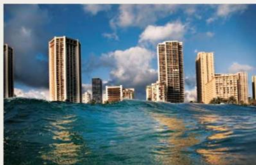
Ocean air: Honolulu will cycle sea water to cool buildings.
